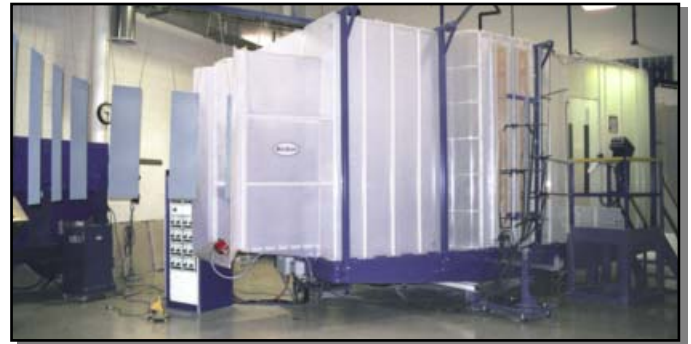
Powder paint facilities.
