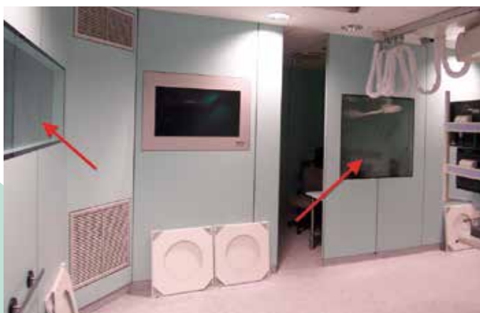
Standard mesh foil mounted with conductive tape 3201
