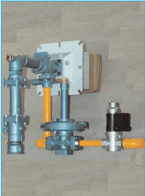
Pre-assembled "Nozzle Mix" burner (Imaformi)
