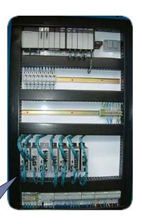
Switches can be either DIN-rail or direct panel mounted
