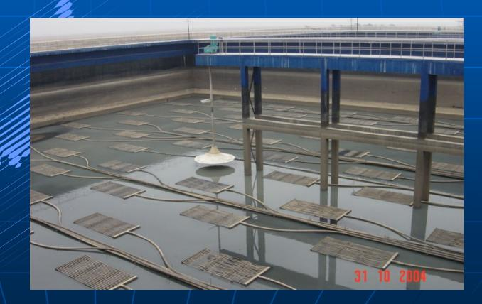
Wear and service parts are not at submersed position. No pull-up of heavy machinery for maintenance.
