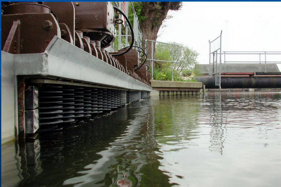
Disc screen for purification of water out of a river (application as cooling water)
