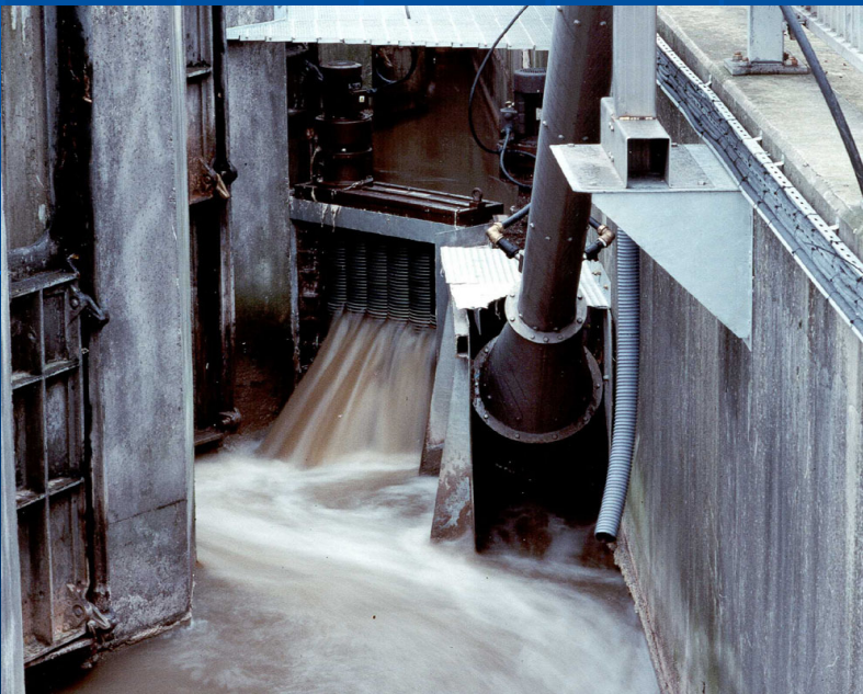
Disc Screen with Muncher and discharge screw
