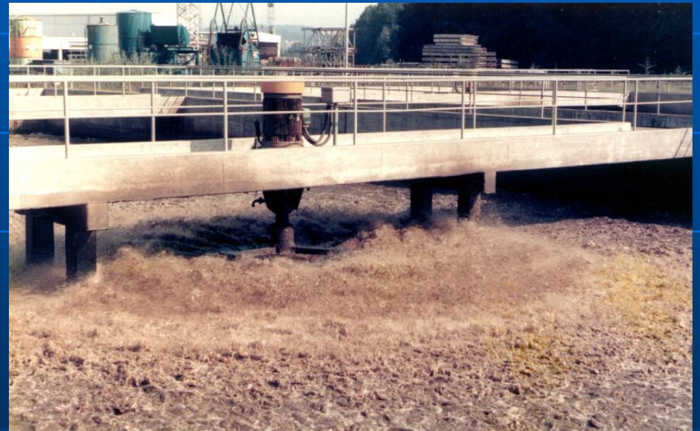
Fixed construction on a bridge (WWTP Luzern – Switzerland)
