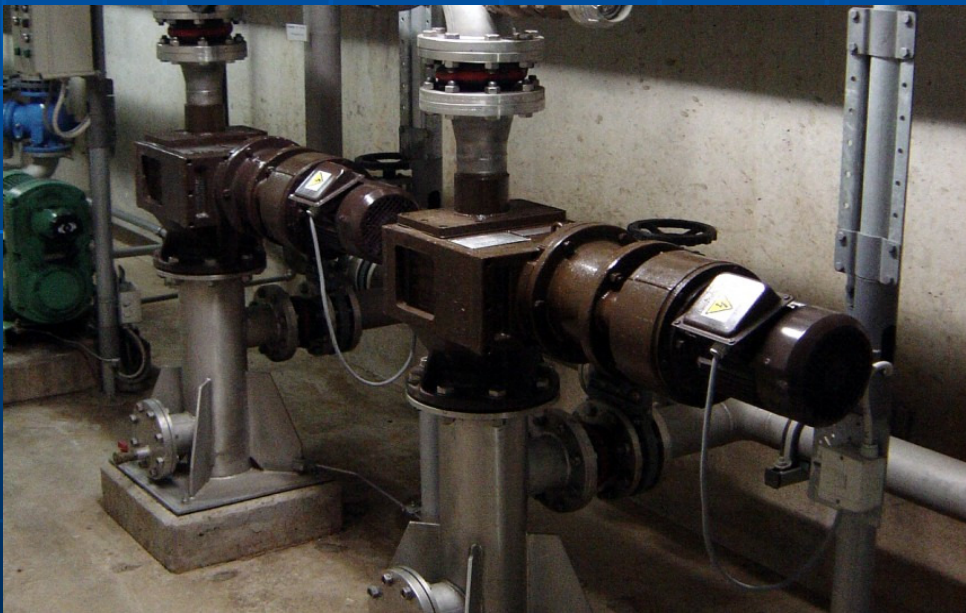
Macerating of solids / fibres containing in the excess sludge of a wastewater treatment plant (before anaerobic digesting)
