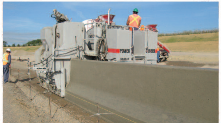
▲ Power Curbers 5700-C Slip-Form Curb Machine
