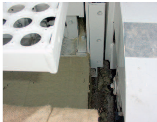
The side-forms are connected to the tracks.
