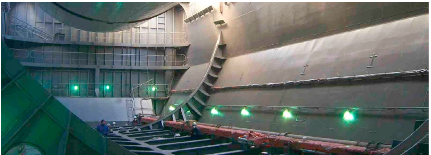
Construction of a liquid gas tank inside a vessel.
