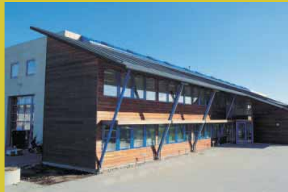
STEMA/PEDAX Headquarters – Denmark
