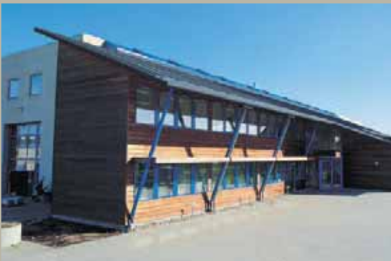
STEMA/PEDAX Headquarters - Denmark
