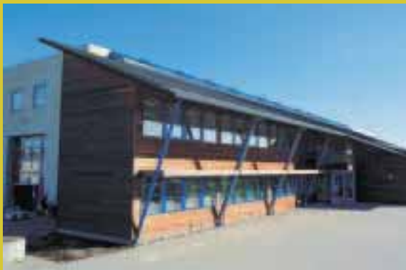
STEMA/PEDAX Headquarters – Denmark
