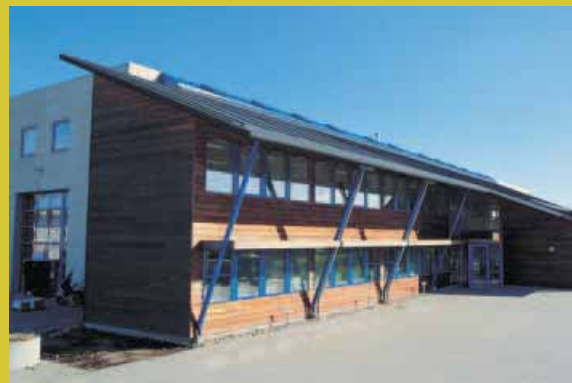
STEMA/PEDAX Headquarters – Denmark
