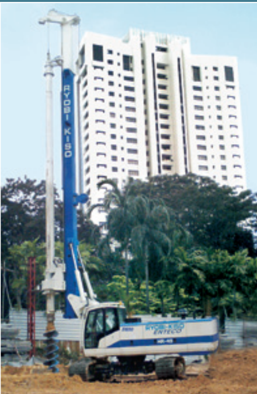
Singapore Edificio commerciale residenziale E6050 – R240 Pali trivellati ø 600-1200 mm. Singapore Housing and commercial complex E6050 – R240 rig model Drilled piles 600-1200 mm.
