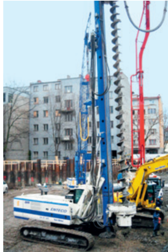
Isola del Tronchetto Venezia (ITALIA) Officina manutenzione natanti pubblici E6050 – SP240 Pali Soil Displacement ø 360-420-520 mm. Tronchetto Island – Venice (Italy) New public transport craft boats maintenance facilities E6050 – SP 240 rig model Soil displacement piles Tools dia. 360-420-520 mm.
