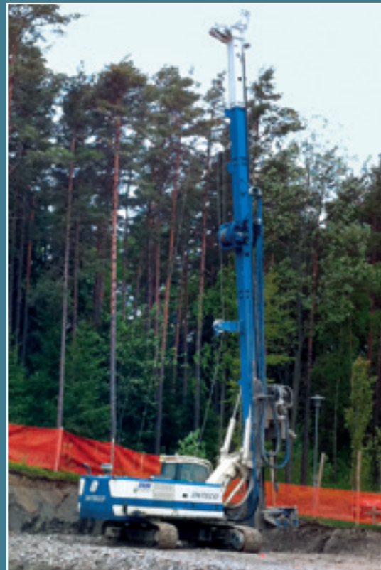
Singapore Edificio commerciale residenziale E6050 – R240 Pali trivellati ø 600-1200 mm. Singapore Housing and commercial complex E6050 – R240 rig model Drilled piles 600-1200 mm.
