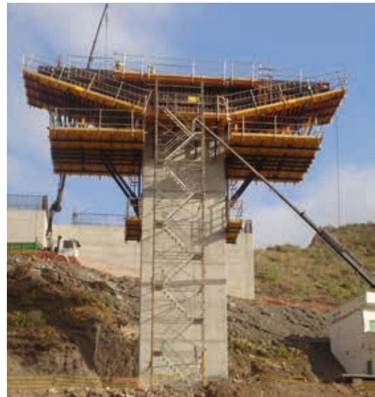
Construction of pier cap with G Bracket
