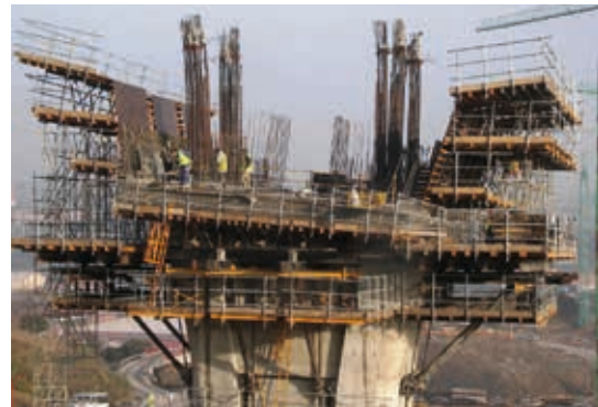
G Heavy duty Bracket in construction of viaduct with superelevation
