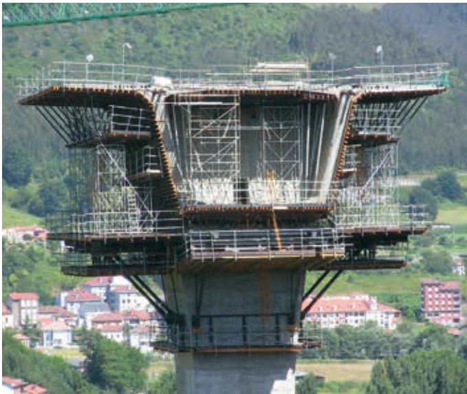
Construction of pier segment
