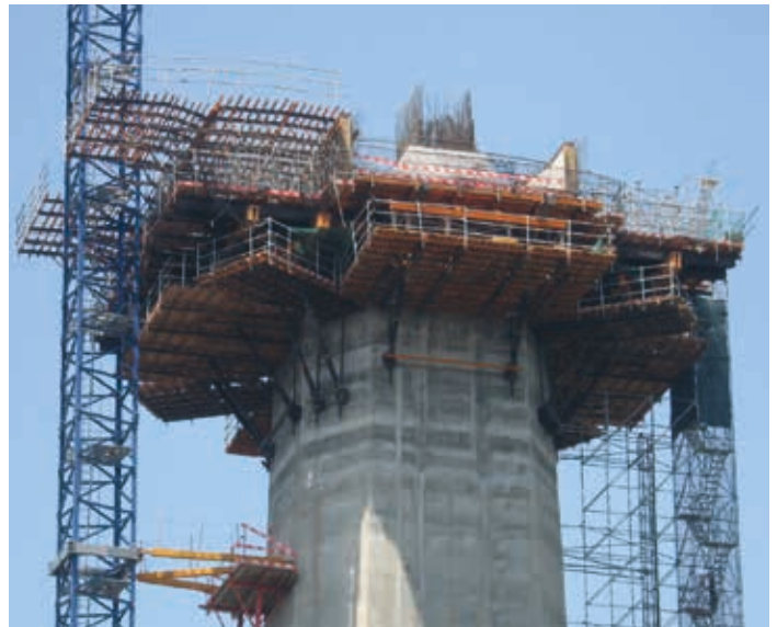
Working platforms in the construction of pier segment
