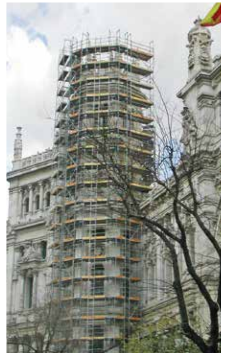
* During the assembly process.
