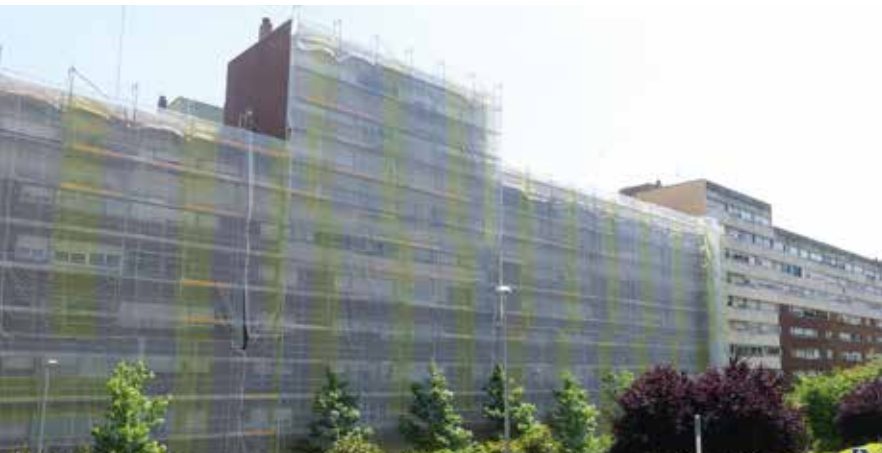
► Building in the Canyelles neighbourhood - BARCELONA
