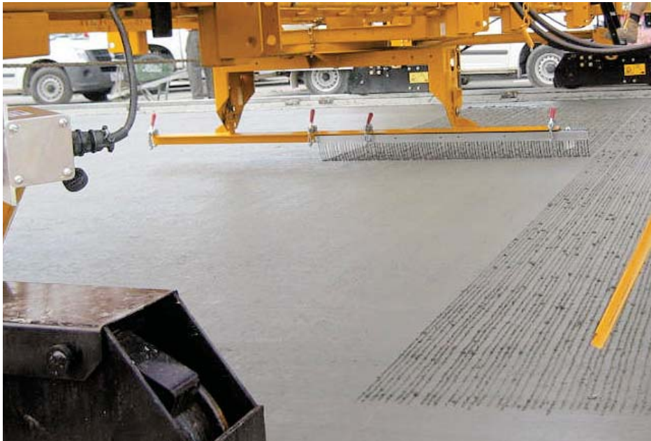
All of GOMACO's texture/cure machines are equipped with a tining bar to apply the proper depth of texture.
