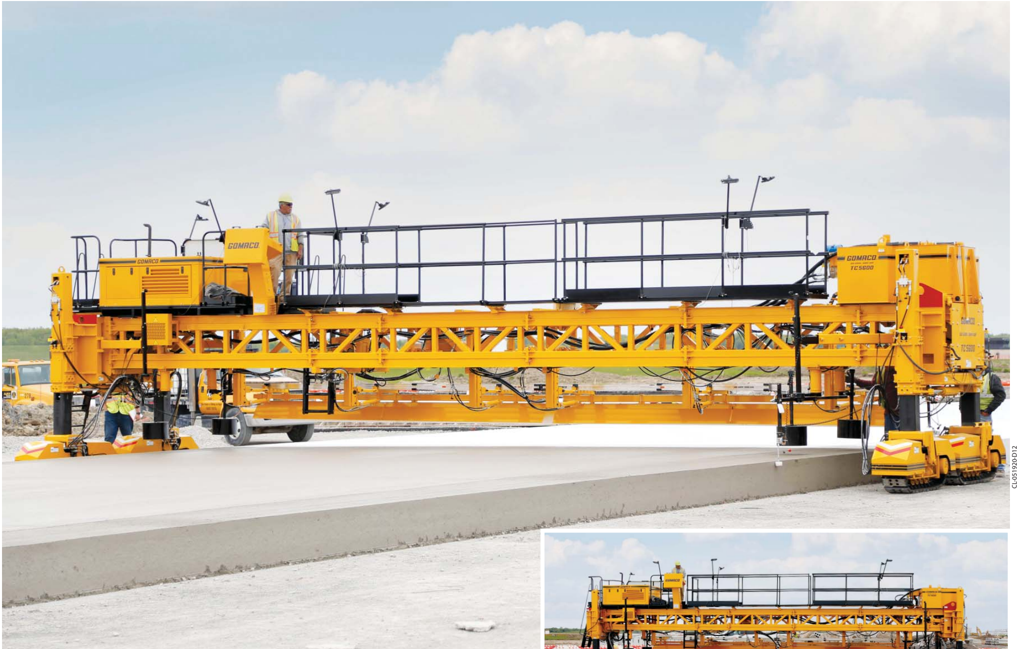
On this airport project, the T/C-5600 is curing 37.5 feet (11.43 m) wide on a new runway (shown above). The contractor was completing multiple paving passes each day and the T/C-5600's ability to turn its tracks 90 degrees allowed it to quickly and easily move from the end of one paving pass to the beginning of the next pass (shown to the right).
