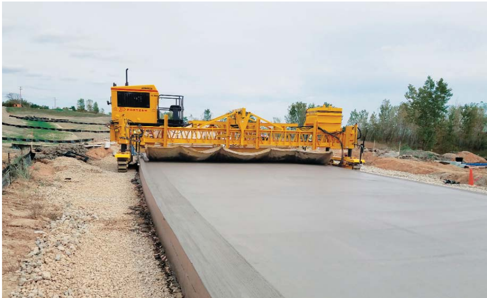
Using poly-wheel sensors for grade and steering off the slab, this T/C-600 texture/cure machine has a burlap drag to texture the new highway per project specifications.
