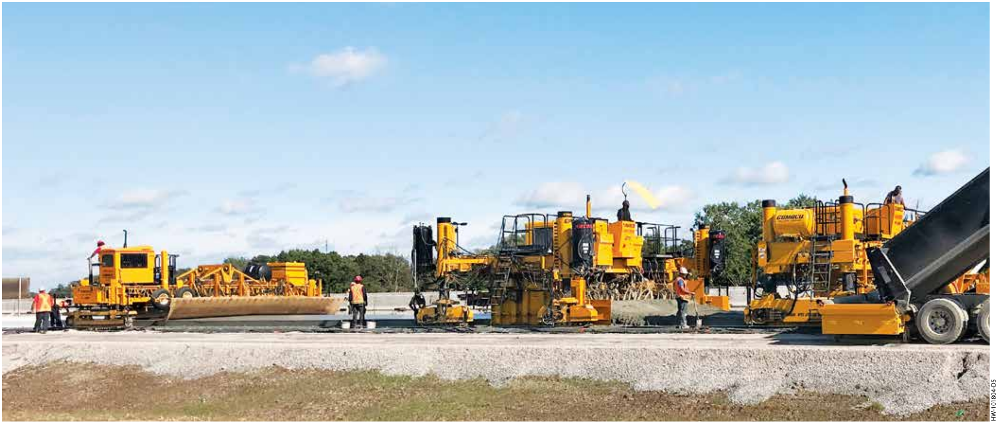
The T/C-600 is applying the texture and cure behind the GOMACO PS-2600 placer/spreader and the GP3 slipform paver on this newly slipformed highway project.
