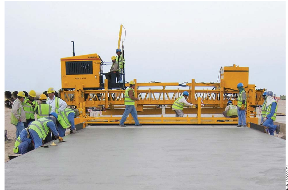
A T/C-400 comes off the header to cure a 19.7 foot (6 m) wide airport apron paving pass on an international airport in Qatar.
