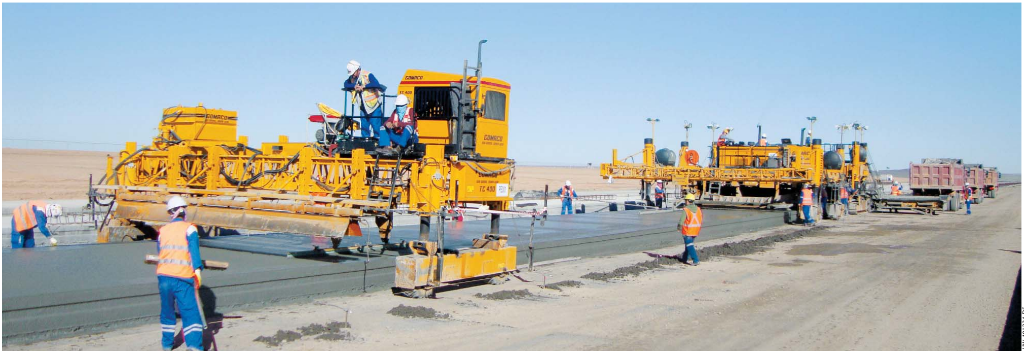
The T/C-400 texture/cure machine uses the optional tining brush to apply texture on this airport project in Mongolia.
