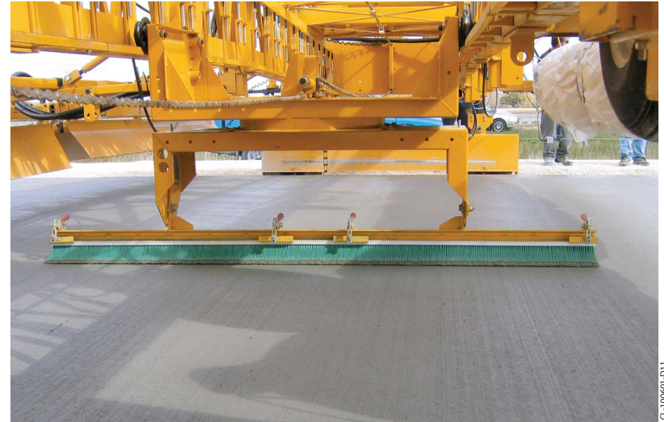
An optional tining brush can be added to GOMACO's texture/cure machines to apply a lighter texture on the surface of the newly slipformed slab.
