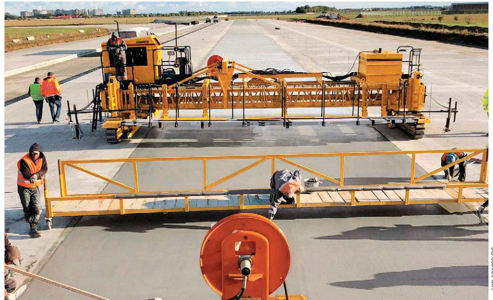
A GOMACO T/C-600 applies the spray cure to the 24.5 foot (7.47 m) wide airport lane at an international airport in the Ukraine.
