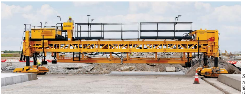
On this airport project, the T/C-5600 is curing 37.5 feet (11.43 m) wide on a new runway (shown above). The contractor was completing multiple paving passes each day and the T/C-5600's ability to turn its tracks 90 degrees allowed it to quickly and easily move from the end of one paving pass to the beginning of the next pass (shown to the right).
