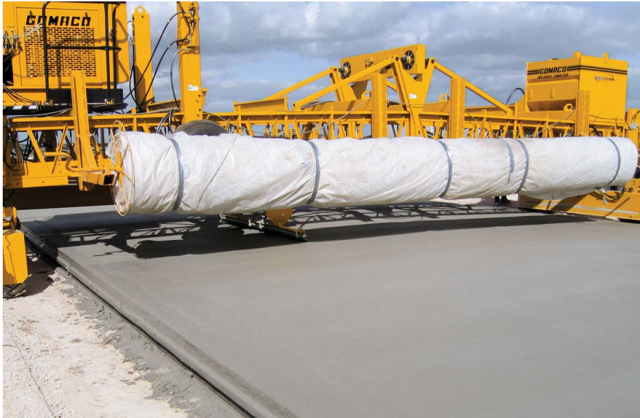
A GOMACO texture/cure machine can be equipped with an optional poly-roll, which can be applied to help protect the slab in the event of rain.
