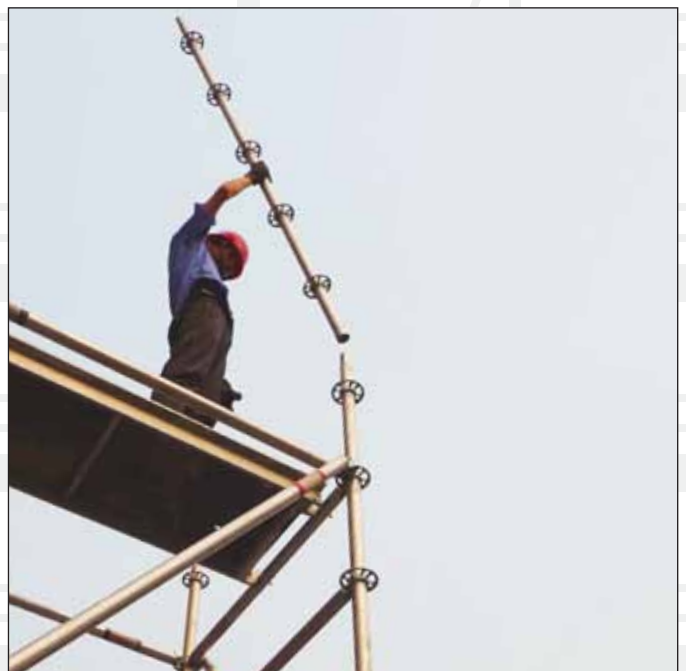
▲ Light weight aluminium components enables fast and labour saving erection of scaffolding.
