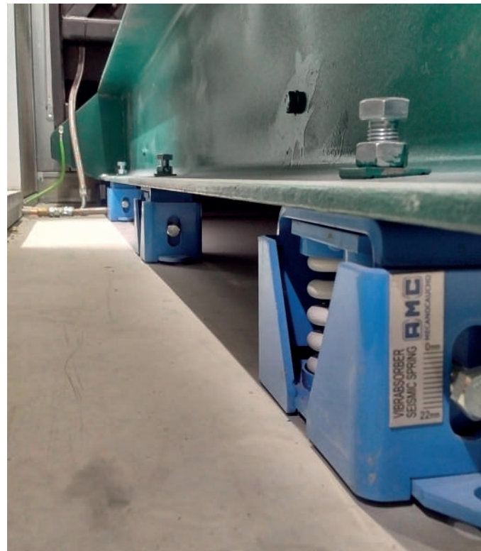
Compressor insulated with VIBRABSORBER +Sylomer®
