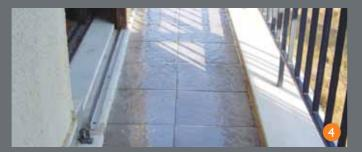
For best results, all surfaces undergoing transparent sealing must be dry and in good condition. Detailed inspection and careful preparation are necessary. Joints and seams must be clean, dry and free of ascending nitric salts deposits. It is recommended that all joints, seams and gaps undergo a pretreatment with a suitable deep penetrating primer. For detailed application instructions please consult the product technical data sheet.
