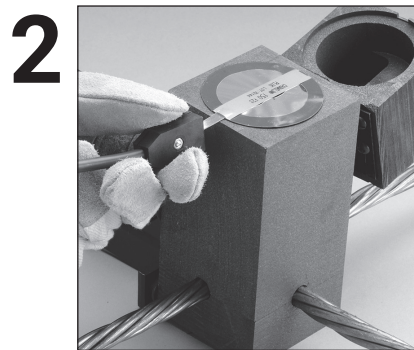
Attach control unit termination clip to ignition strip
