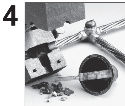
Open the mold and remove the expended steel cup – no special disposal required
