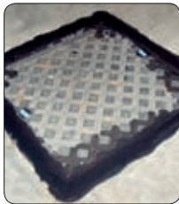
Scellage des cockpits
