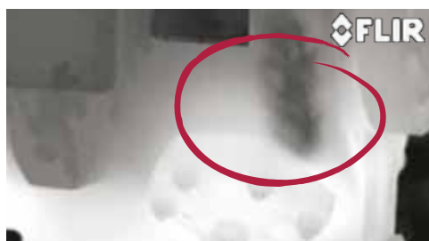
Captured gas leak.
