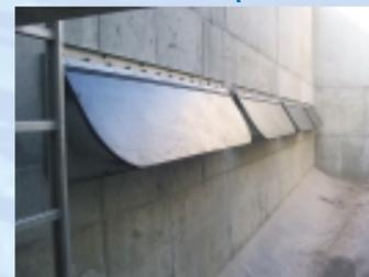
Clapet anti-retour FluidSlot
