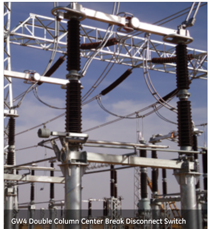
GW4 Double Column Center Break Disconnect Switch
