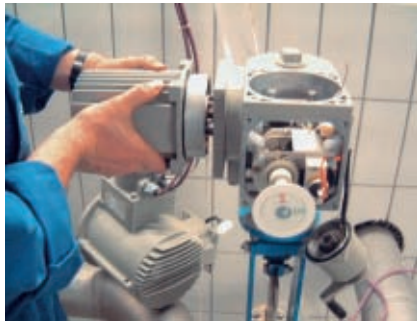
Inspection in fine detail
