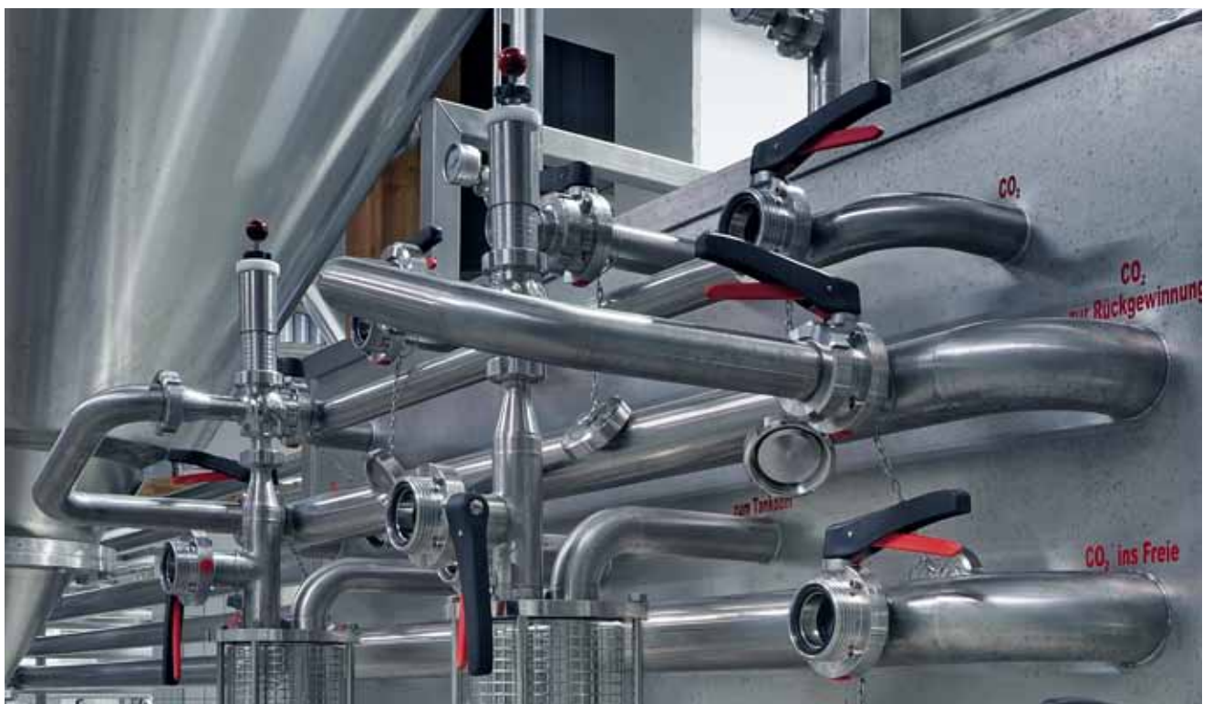
Panel with bunging valves in a brewery
