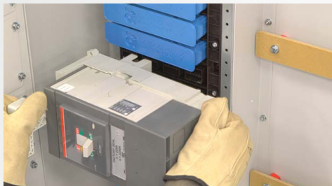
The Breaker Is Inserted Into The SafePanel
