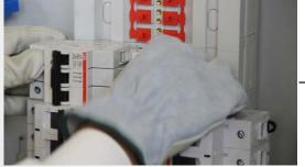
The Breaker Snaps Into The DIN Rail
