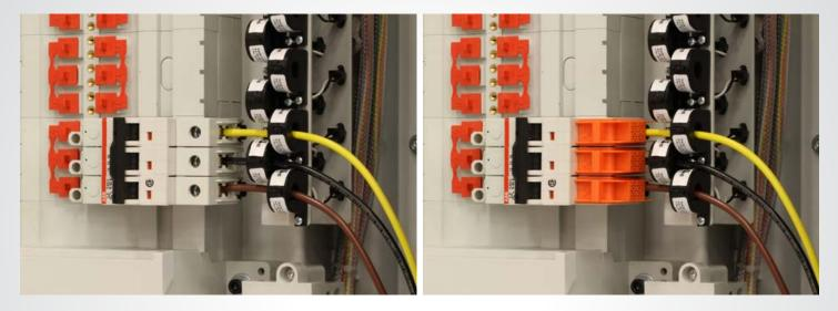
Wiring Without Shrouds Leaves Wiring Exposed
