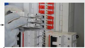
The Breaker Is Inserted Into The Opening
