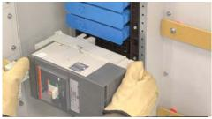
The Breaker Is Inserted Into The SafePanel
