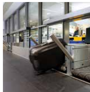
The belts are so flat and smooth that transferring items onto the conveyor from the sides is no problem.
