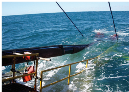
Smart ® Band installed on Piggyback Pipelay operation
