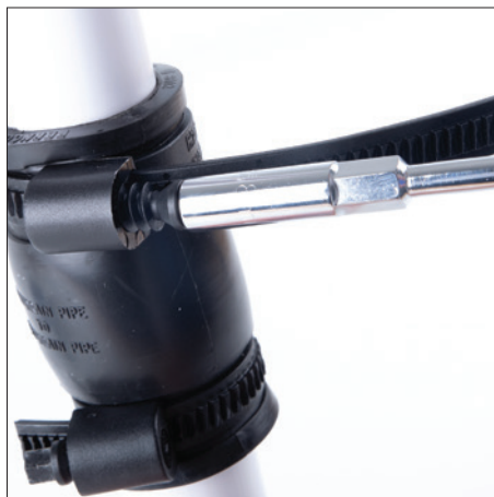
Tighten using Manual 8mm Hex Screw Driver
