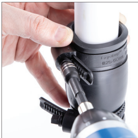
Tighten using Electric Screw Driver
