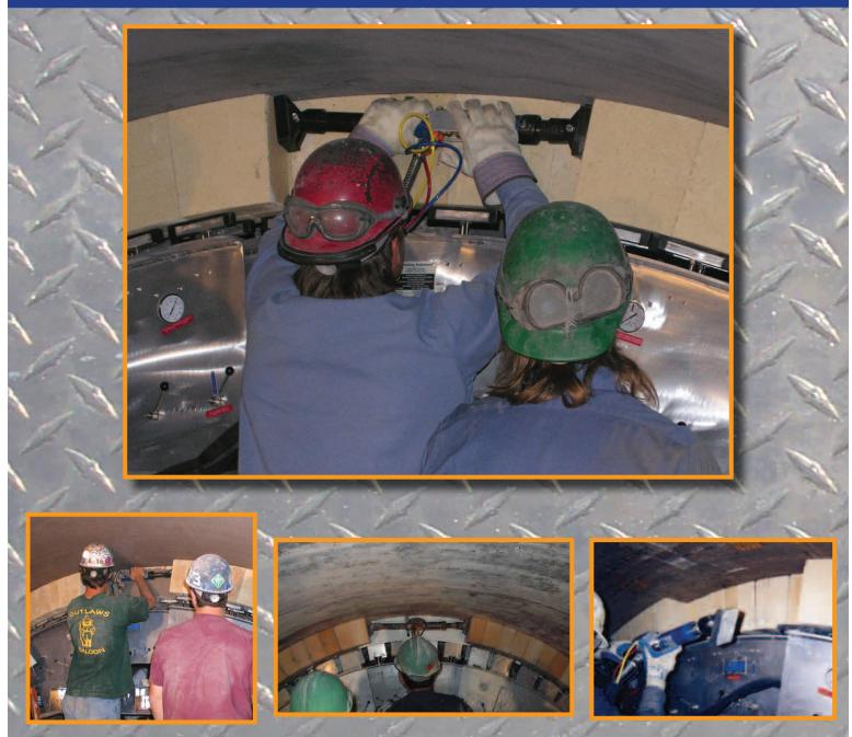
The Long Jack uses finger tip controls to make installing each course of brick easier and faster
