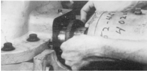
FIGURE 18 - INSERTING PACKING INTO STUFFING BOX
