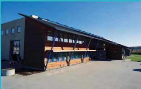
STEMA/PEDAX Headquarters - Denmark
