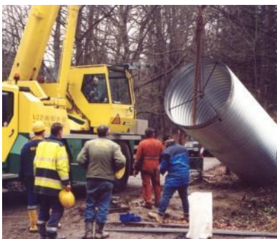
Displacement pipe ø 1.8 m for ventilation shaft in tunnel construction
