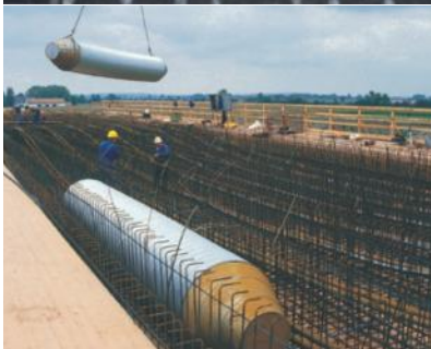
Installation of displacement pipes at a bridge construction site
