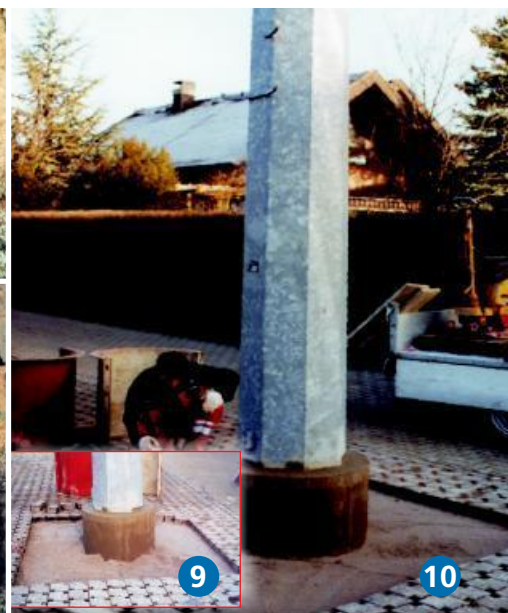
Example of use: Electricity pylon foundations, photos 5 to 10
