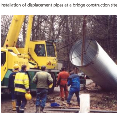
Installation of displacement pipes at a bridge construction site
