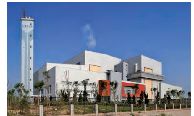
◇ Qingdao Xiaojianxi Municipal Solid Waste (MSW) Incineration Plant (China) / Realizes low NOx and dioxin emission reduction.
