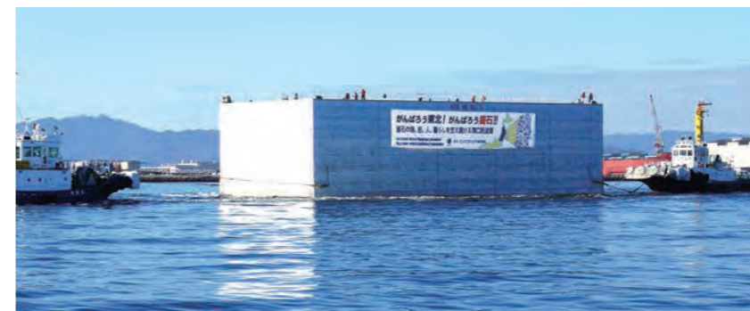
◇ Kamaishi Port Breakwater (Iwate Pref.) / Hybrid Caisson of the breakwater entrance during towing
