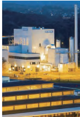
◇ Lünen Biomass Power Plant (Germany)
