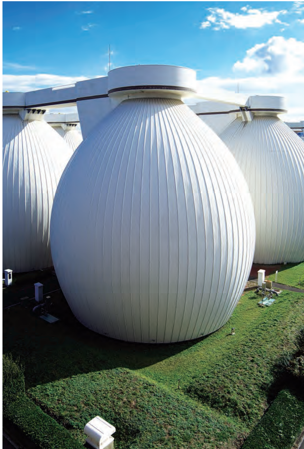
◇ Sewage sludge digestion gas power generation facility (Kanagawa Pref.)
