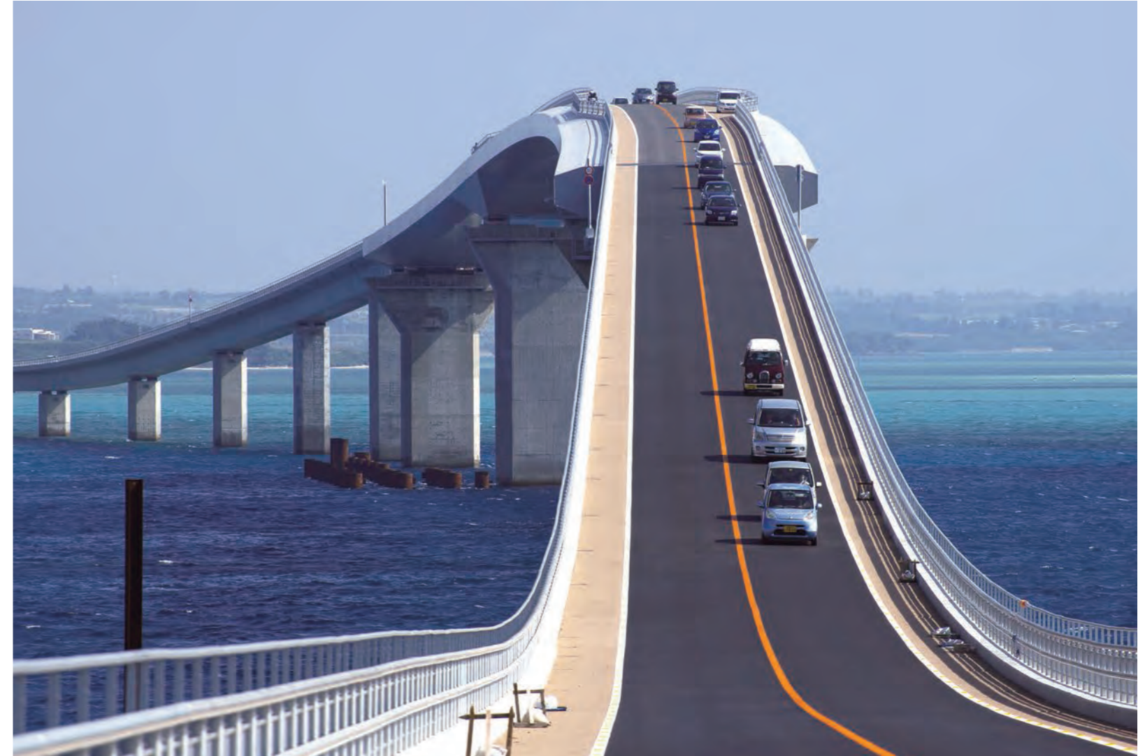
◇ Irabu Bridge (Okinawa Pref.) / A huge bridge girder block with a total length of 140m and weight of 1,300t, which was fabricated in JFE's Tsu Works, was erected in only 1 day.
