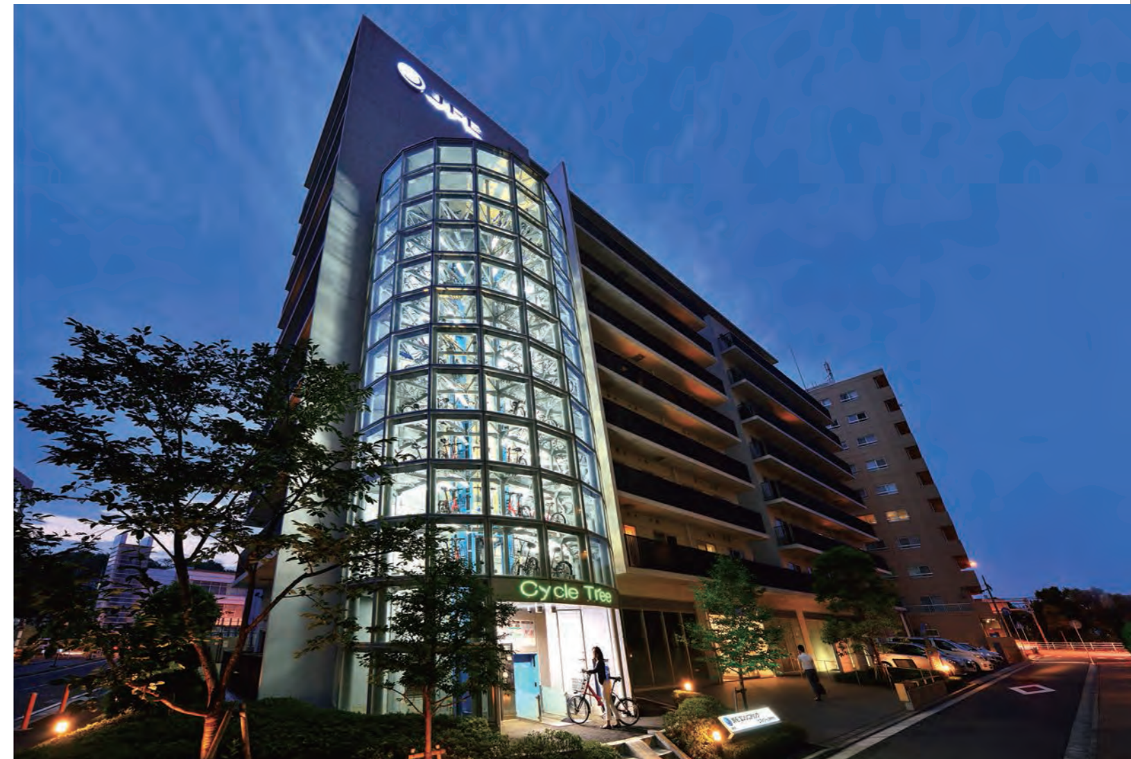
◇ JFE Engineering’s “Cycle Tree” (mechanical multilevel bicycle parking system) can store bicycles efficiently (Kanagawa Pref.) / The winning solution for the problem of bicycles left around train stations.
