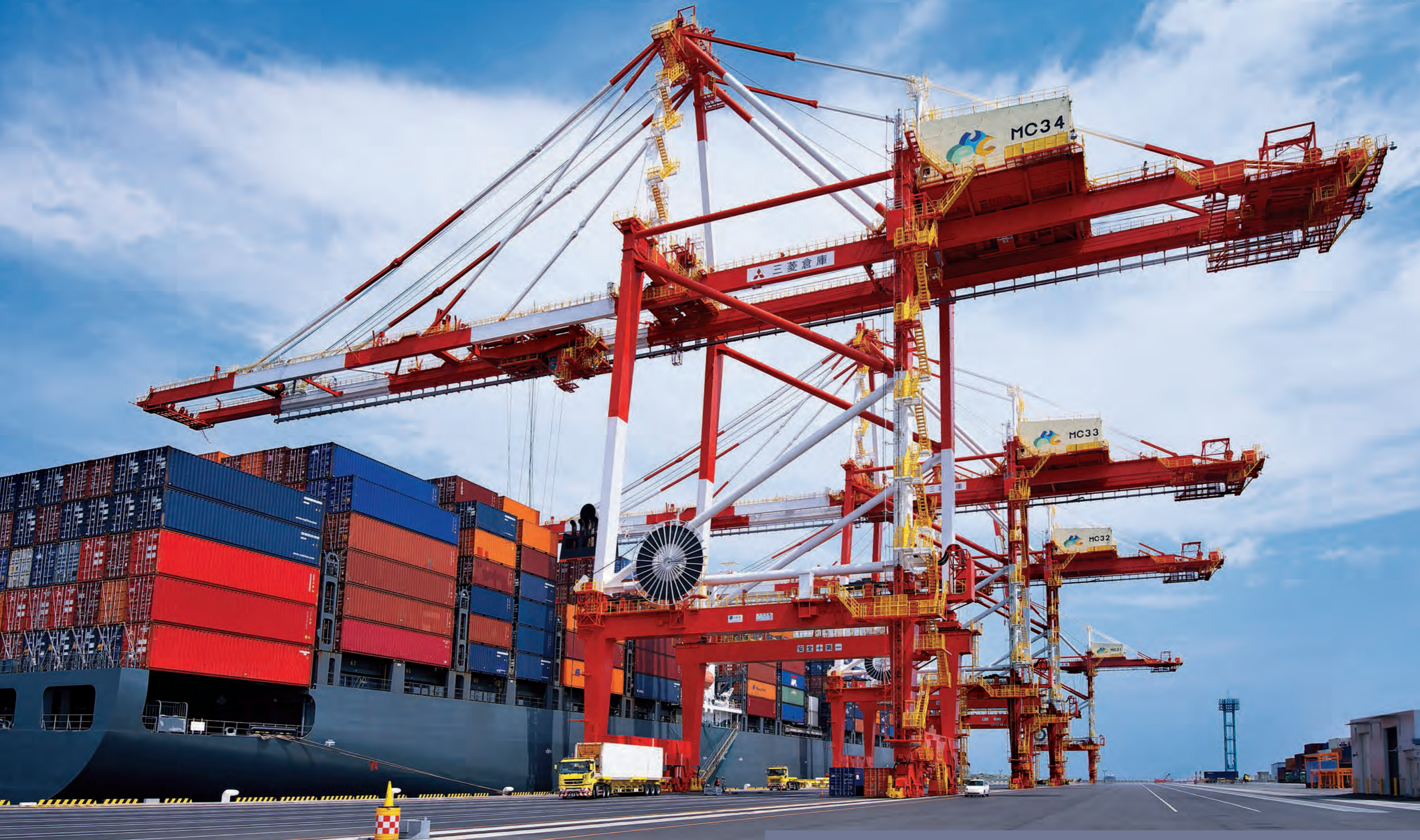
◇ Container cranes at the Port of Yokohama, Minami Honmoku (Kanagawa Pref.) / The world's largest seismic-isolated cranes are playing an active role in improving cargo-handling in the Port of Yokohama.
