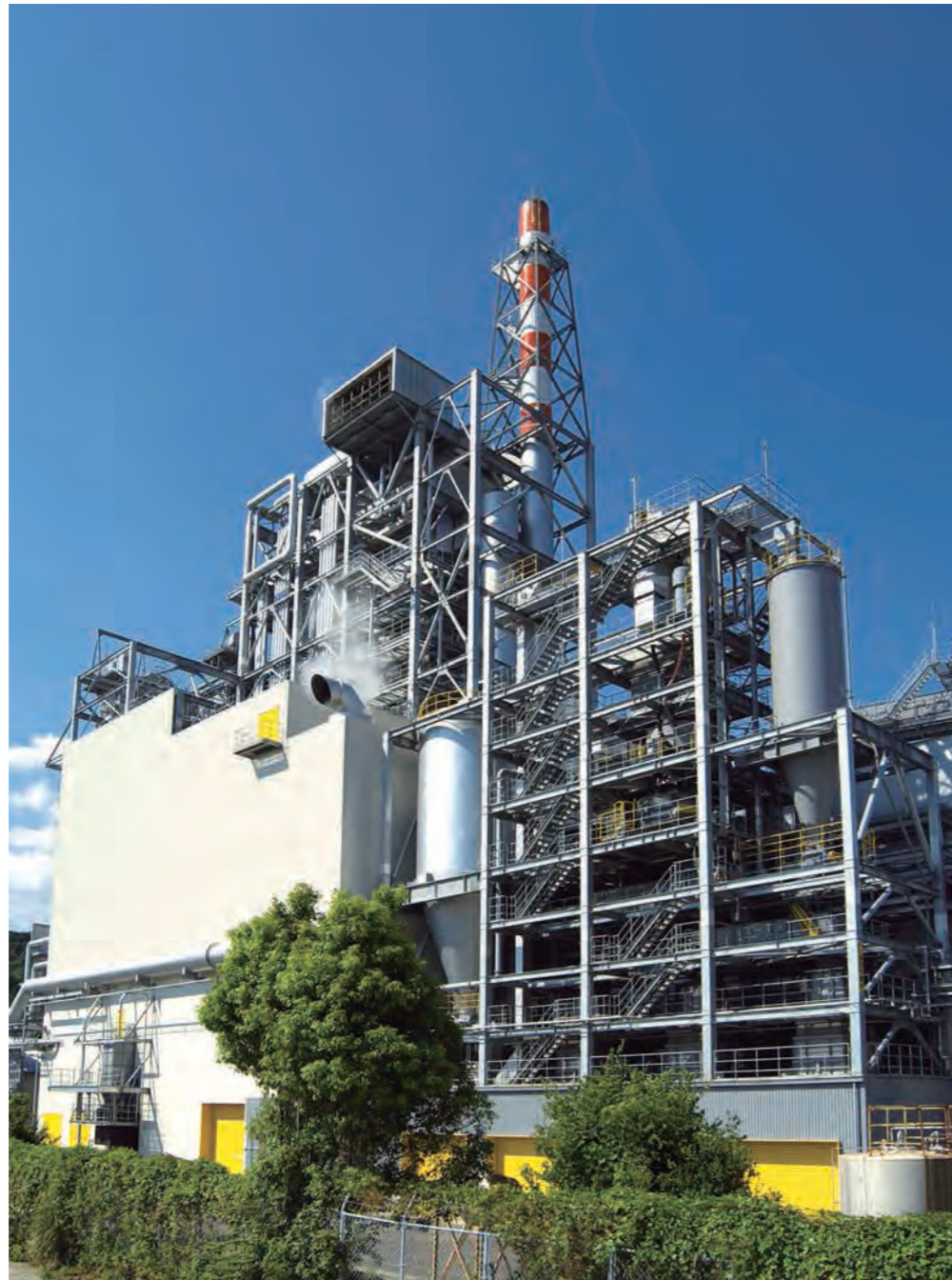
◇ Biomass boiler at Hokuetsu Kishu Paper Co., Ltd. (Mie Pref.)
