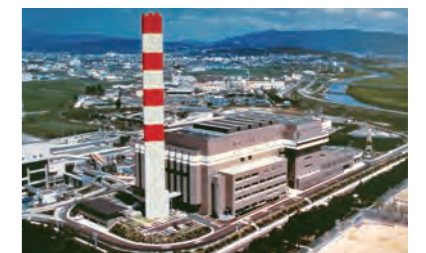
◇ Kyoto Minami Waste Incineration Plant (1983)
