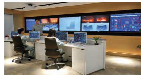
◇ Remote Service Center (JFE Engineering Yokohama Head Office) / Centralized management of the operating condition and power generation status of waste to energy plants by a 24-hour-day system.
