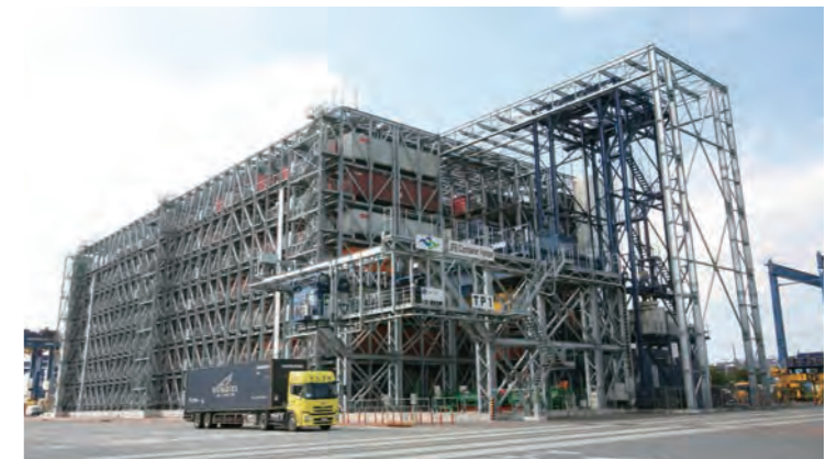
◇ Oi Wharf multilevel container warehouse (Tokyo)
