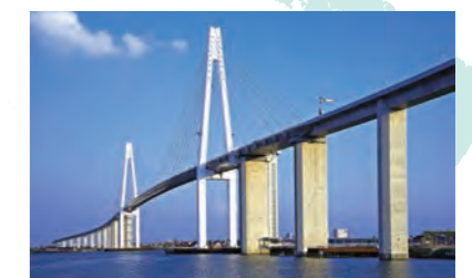
◇ Shinminato Bridge, Toyama Pref. (2011)
