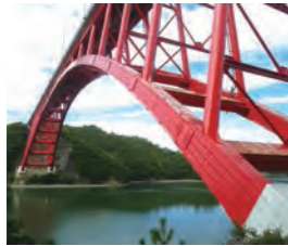
◇ Matoya Bay Bridge (Mie Pref.)
