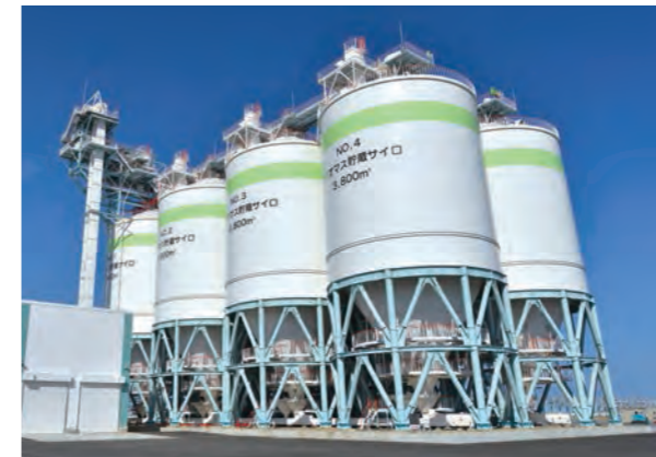
◇ Biomass silos (Ibaraki Pref.) / Japan’s largest wood fuel storage and conveying facility.
