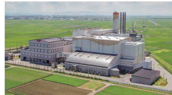
◇ Shinden Refuse Incineration Center (Niigata Pref.)
