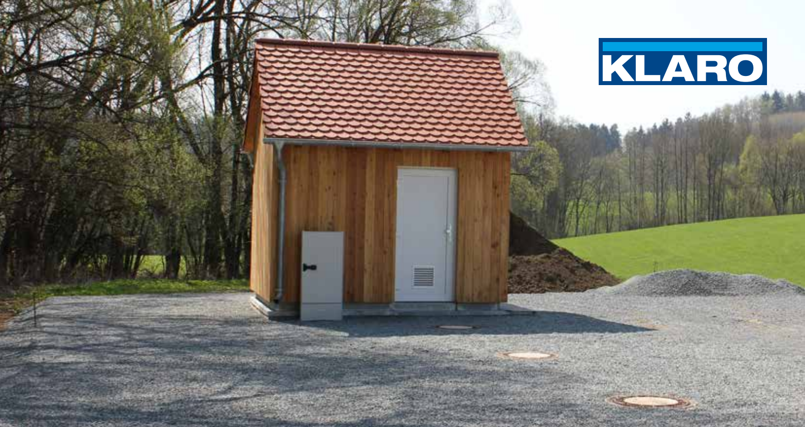
Machine cabin of a 100 PE plant
