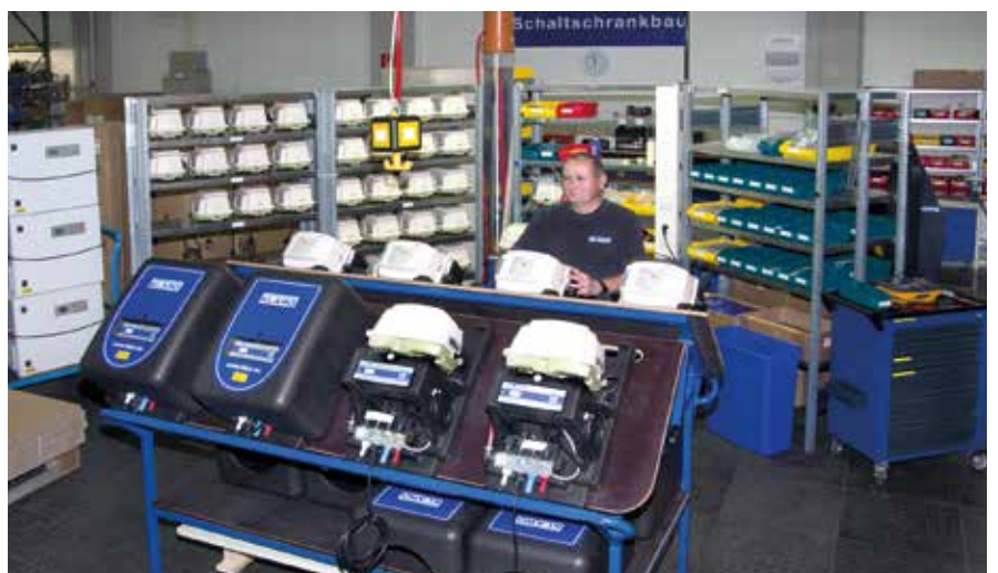
switch cabinet production
