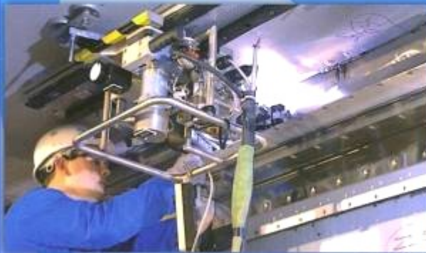
ERI automatic welding machine ceiling position
