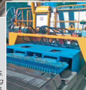
PRESLABS. Slipforming process.
