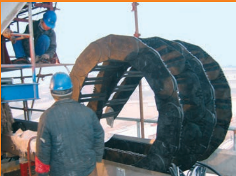
Installation of an E4.1 e-chain® Series 800 in an igus® steel guide trough
