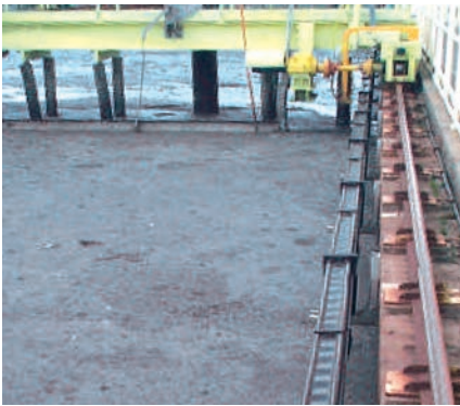
igus® lbt flizz® - Sewage works of the company Hydrobudowa S.A. in Poland. The power supply system of the scrapers in 8 clarifiers was equipped with igus® e-chain® and lbt flizz®. The complete system runs directly over the clarifier. Advantages: ● Low-maintenance system ● Longer service life ● Enclosed trough, protection against snow and ice ● Space-saving compared to conventional system ● Compact and safe ● Travel (S) = 42 m ● Assembled with igus® chainflex® cables
