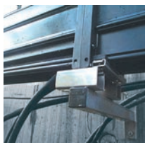
Example of mounting the console on jibs
