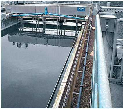
lbt flizz® in a longitudinal scraper travel (S) = 38 m ● Speed (v) = 1.0 m/min. ● Acceleration (a) = 0.5 m/s 2 ● Cycle time 1.5 x hour/ 24 h/365 days
