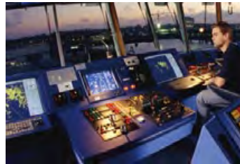
Multiple Control Displays
