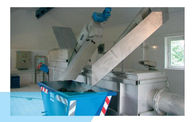
Complete Plant with integrated cross-flow lamella separator
