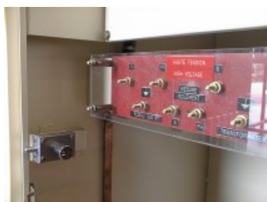
Plaque de Raccordement 3200 V
