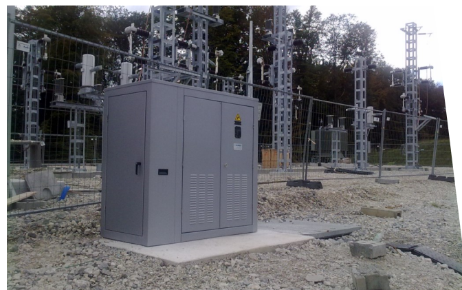
LGV Rhin Rhône, alimentation instrumentation
