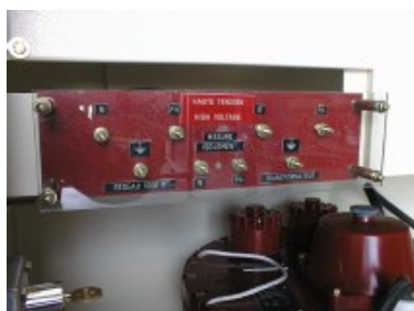
Plaque de Raccordement 3200 V
