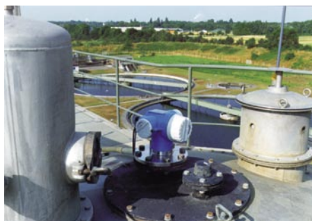
FMR 230 foam detection using radar level measurement
