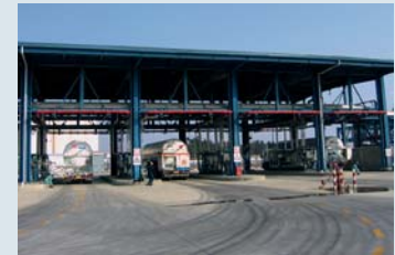
Loading bay management
